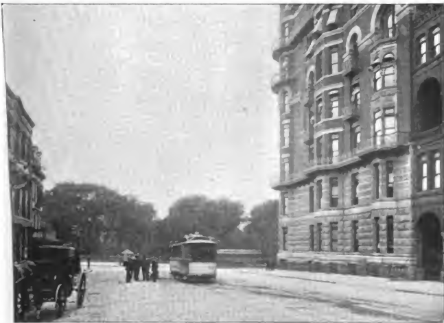
CENTRAL PARK ENTRANCE, AT SEVENTH AVENUE AND 59TH STREET.
